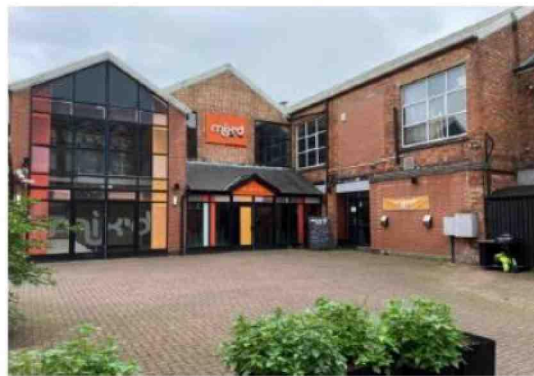
Figure 3: Existing front elevations at 73b Church Gate
