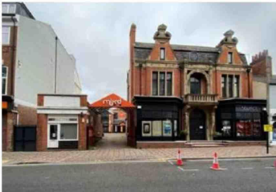
Figure 2: Access to site from Church Gate
